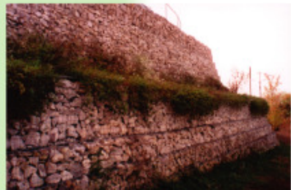
Claycomo, Missouri, USA - retaining wall planted with indigenous ground cover
