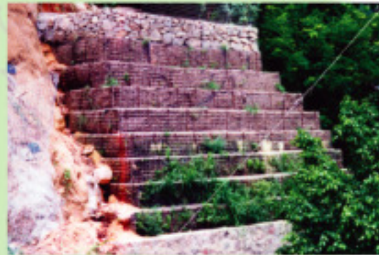
Acapulco, Mexico - revegetated retaining wall
