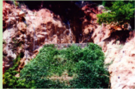
Acapulco, Mexico - revegetated retaining wall
