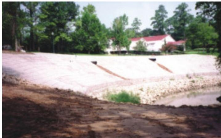
**gabion mattress** *n.*, - a gabion with relatively small height in relation to the lateral dimensions, generally used for lining channels, bank and shore protection, levee revetment, scour protection aprons, etc.
