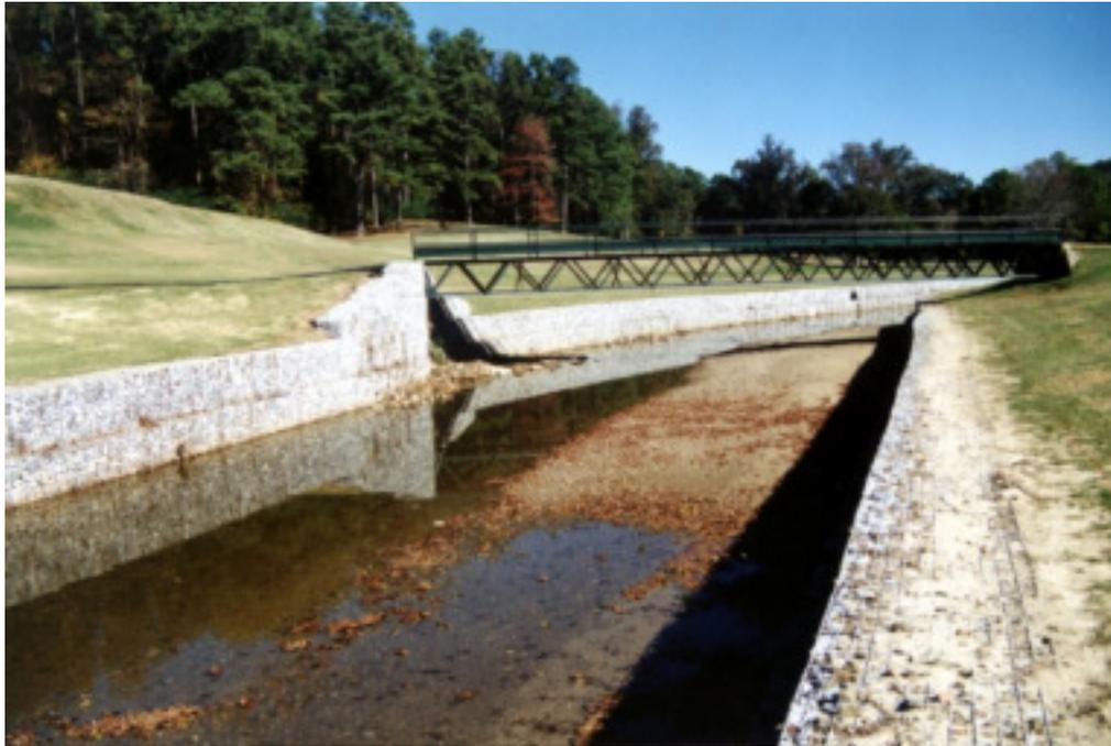
Modular Gabions & Gabion Mattresses conform to ASTM A 974-97 and are ideal for:
